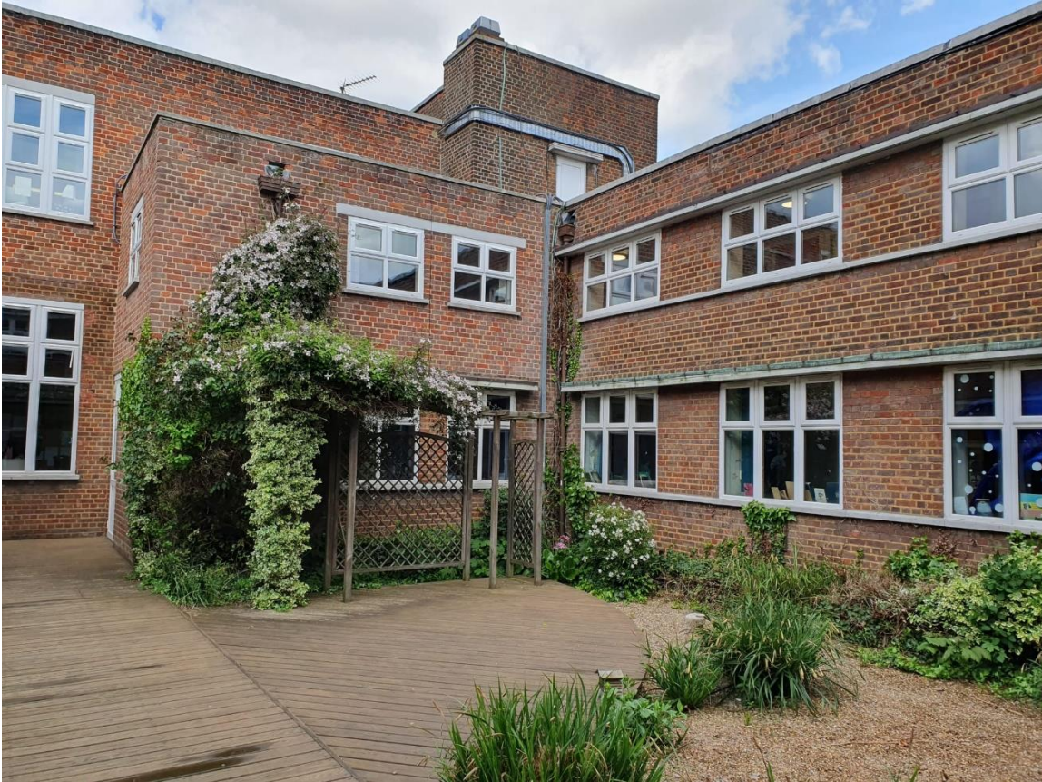
View of Courtyard and Protruding Element:
