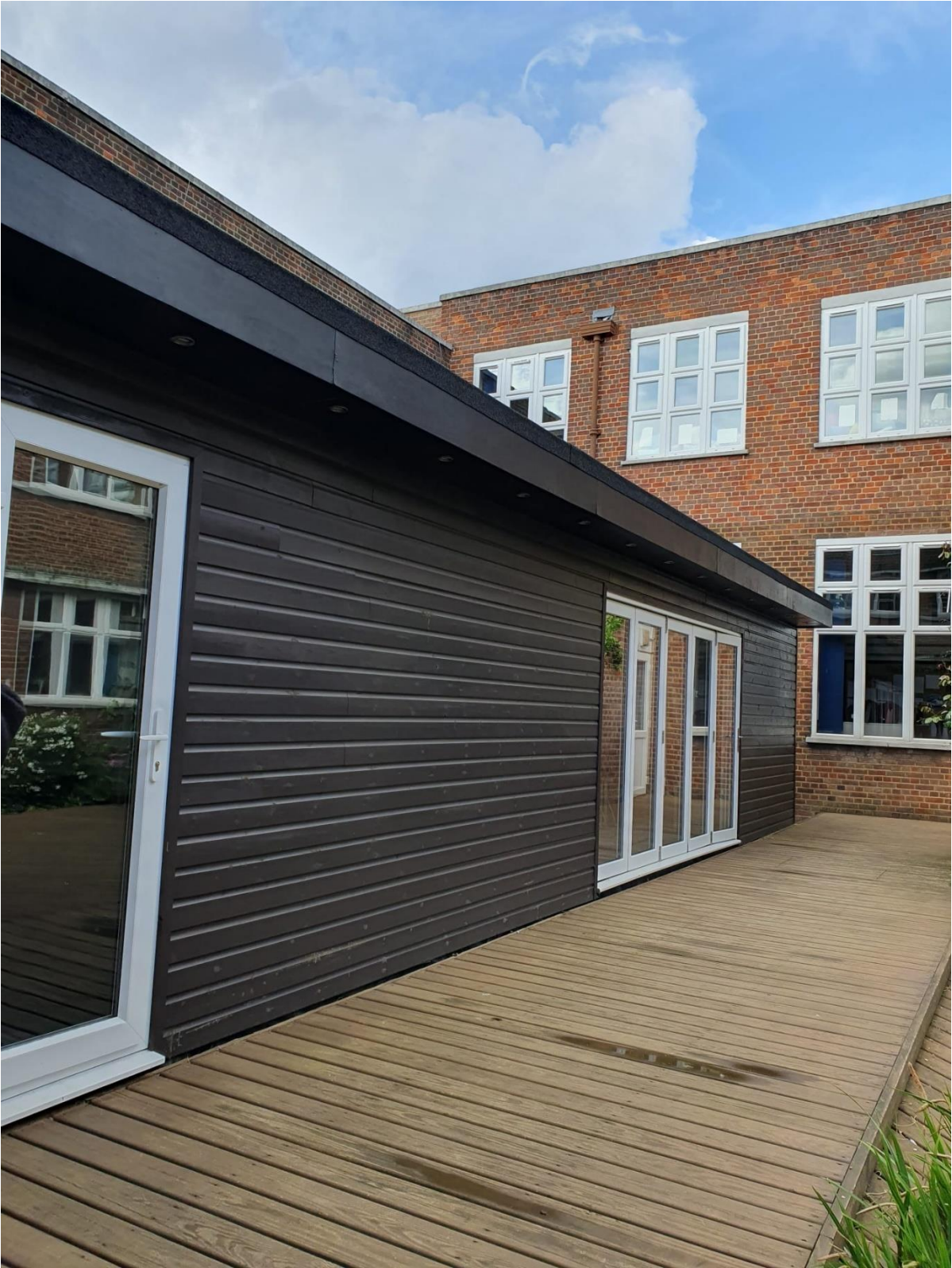
View of Timber Outbuilding:
